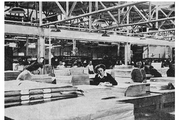
A PORTION OF THE FINISHING ROOM
